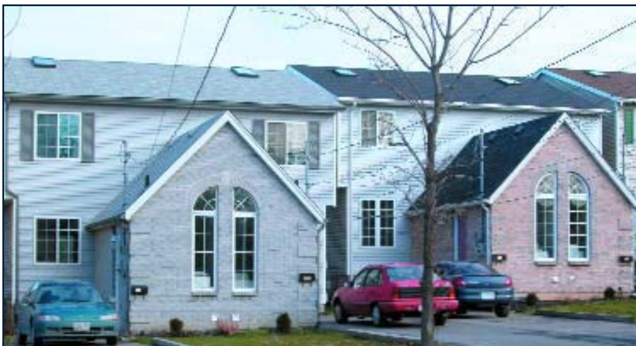
Dr. Tony Shaw of Brock University compared the thermal efficiency of two units in these nearly identical semi-detached homes. The house on the left was built with SIPs, while the other was framed with studs and batt insulation.
